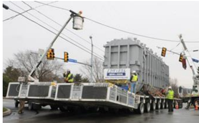
Figure 4. Transport of Large Power Transformers
